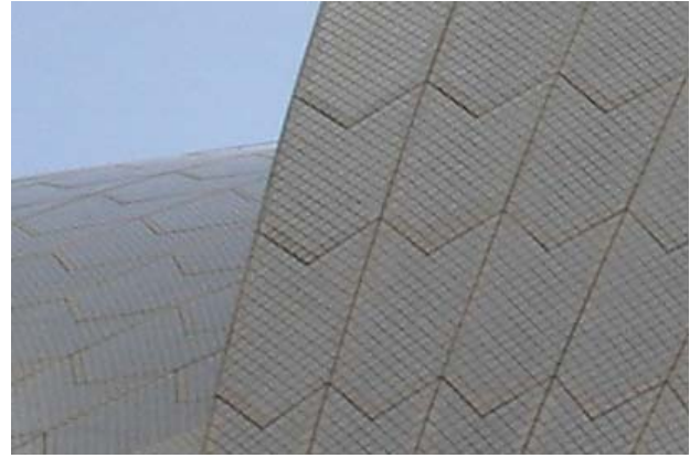
The ceramic tiles were fabricated on the ground in the chevron shaped modules and then installed on the structure.
