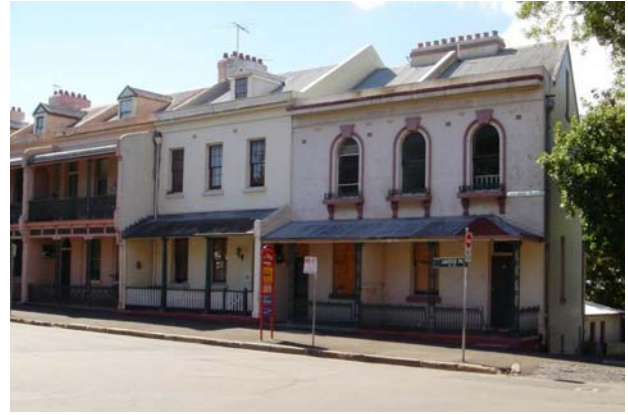
The first houses built in the Rocks. They were packed in like sardines.
